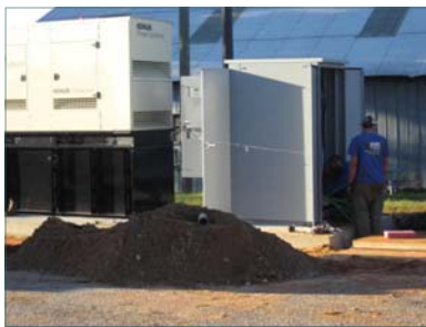
Workers prepare to connect a new emergency generator to the electrical system of Building 76 on the Gracewood Campus.
