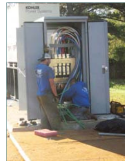
Workers prepare to connect a new emergency generator to the electrical system of Building 76 on the Gracewood Campus.
