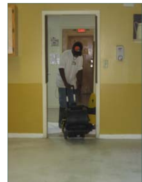
Putting a shine on the new floor in House 3 on the Gracewood Campus.
