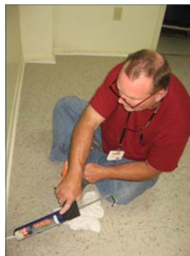
Carey Smith caulks the baseboards after the new floor was installed in House 3.
