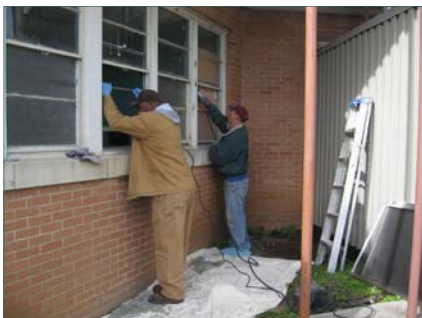
Plant Operations replacing windows as they transform an activities room into a bedroom.
