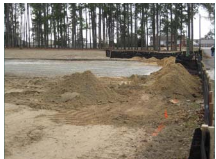
City of Augusta Utilities Department is replacing an 8-inch water line on North Campus.
