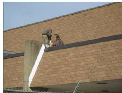
Contractors do some spot repairs to the gym roof on the Augusta Campus.
