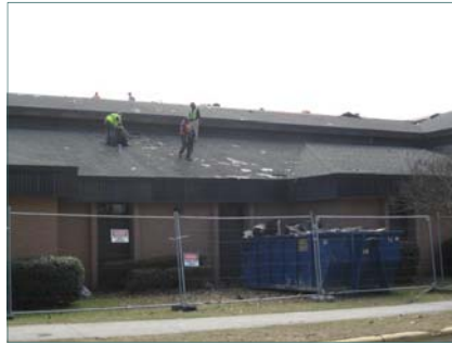
Workers continue to replace the roof on Building 15 on the Gracewood Campus.
