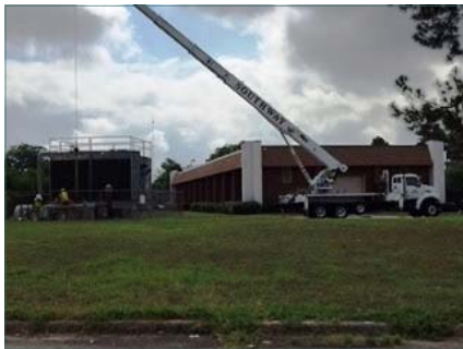
Working on the boilers at the Steam Plant.
