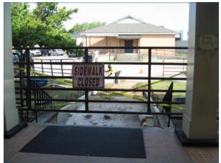
Putting in a new ramp at Building 76.
