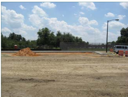
Progress continues on the new parking lot at AMH.
