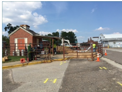
Getting those pesky steam leaks fixed.
