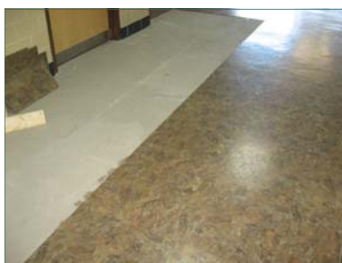
New floor covering being installed in the Camellia Unit.
