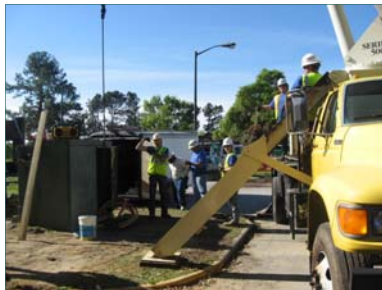
Workers continue to install new emergency generators.
