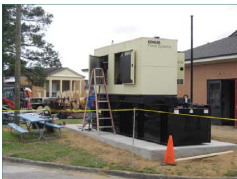
A new generator for Redbud Unit is being installed.
